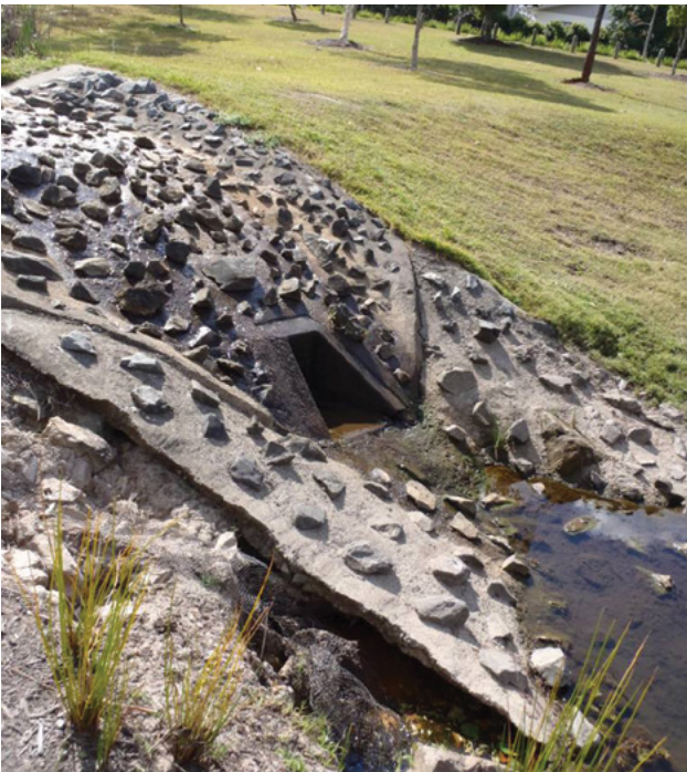
Photo: Colin Bridges, Gold Coast City Council
