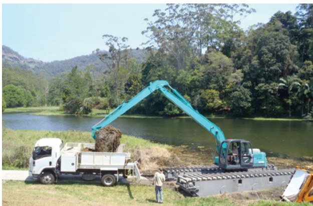
Photo: Colin Bridges, Gold Coast City Council
