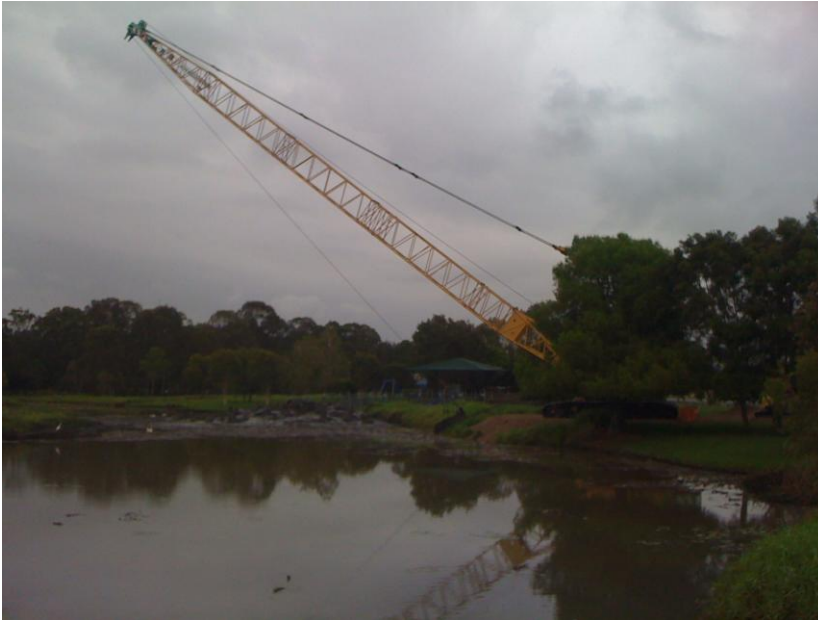
Plate 3 Sediment removal from an urban lake in Brisbane
