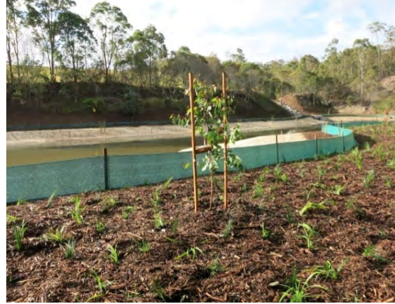
Figure 3.9 Sediment control fence around a constructed wetland.
