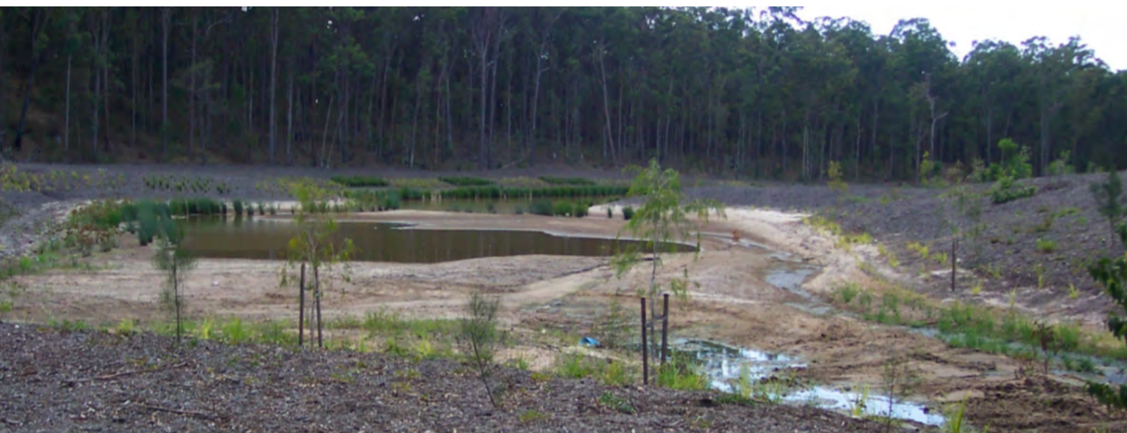
Figure 3.13 Use of a constructed wetland as a HES basin during the building phase.
