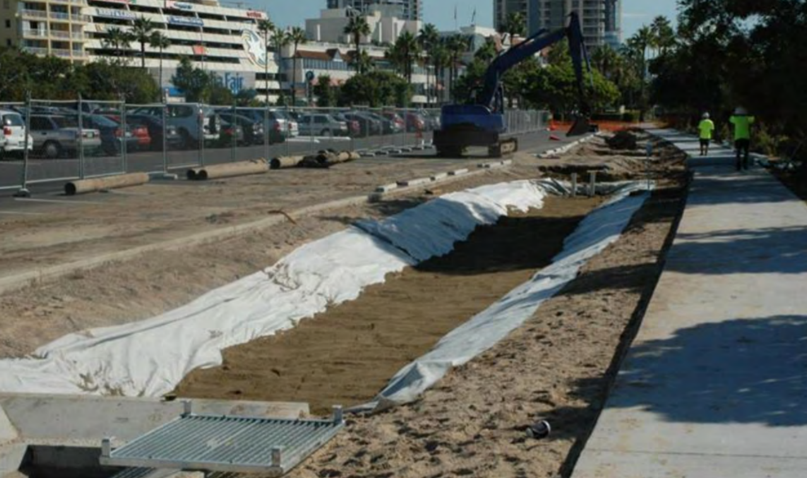
Figure 2.32 Installation of the filter media in a bioretention system.
