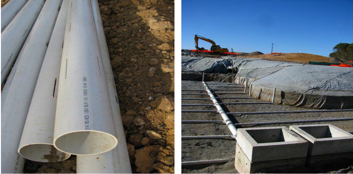
Figure 2.4 Under-drainage pipes in a bioretention system.
