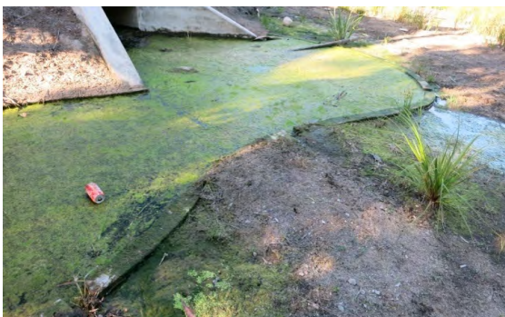
Figure 2.10 Build up of algae and sediment downstream of a coarse sediment forebay.
