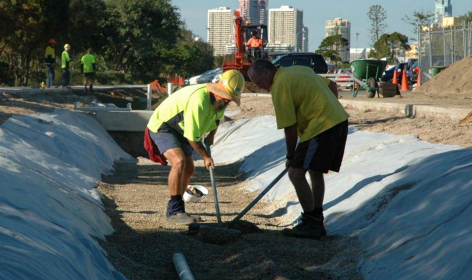
Figure 2.31 Installation of drainage layer materials in a bioretention system.
