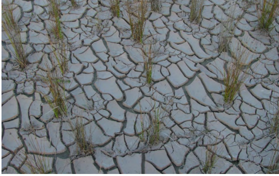
Figure 2.20 Sediment from construction phase activities in a bioretention system.
