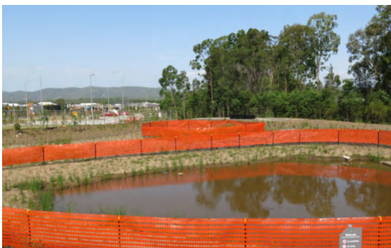
Figure 3.20 Temporary sediment fencing around a constructed wetland.
