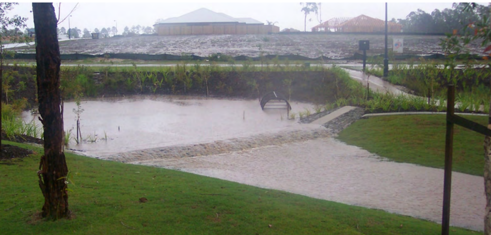
Figure 3.14 Macrophyte zone disconnection in a constructed wetland.
