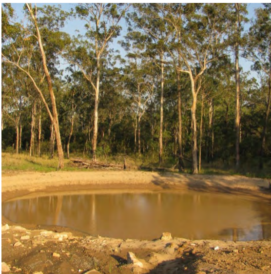
Figure 3.18 Use of a constructed wetland as a HES basin during the building phase.
