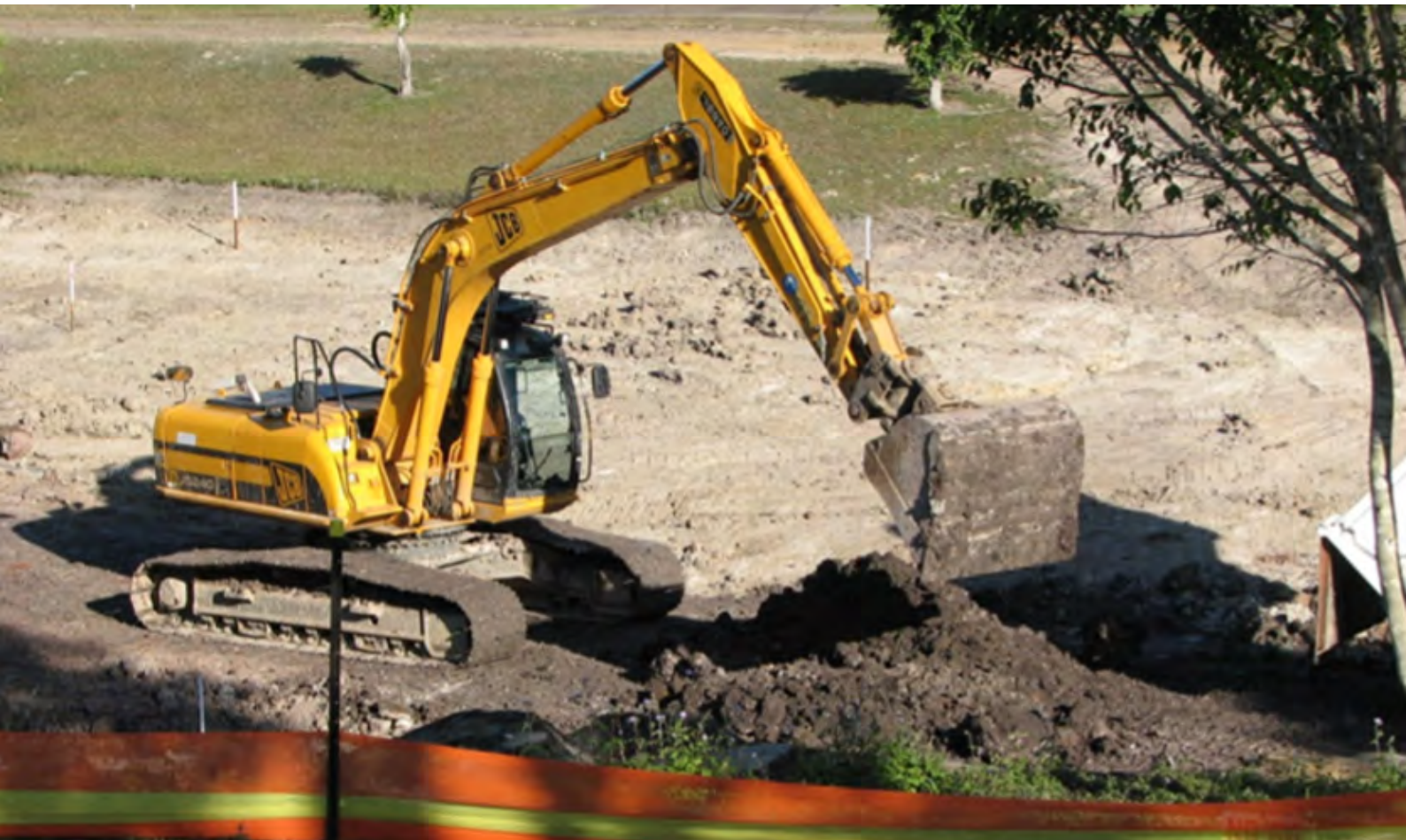
Figure 3.15 Excavator stripping back topsoil in a constructed wetland.
