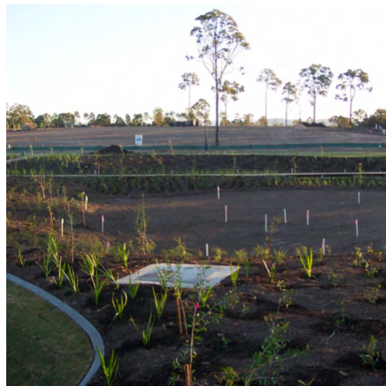
Figure 3.19 Finished surfaced level of a constructed wetland.
