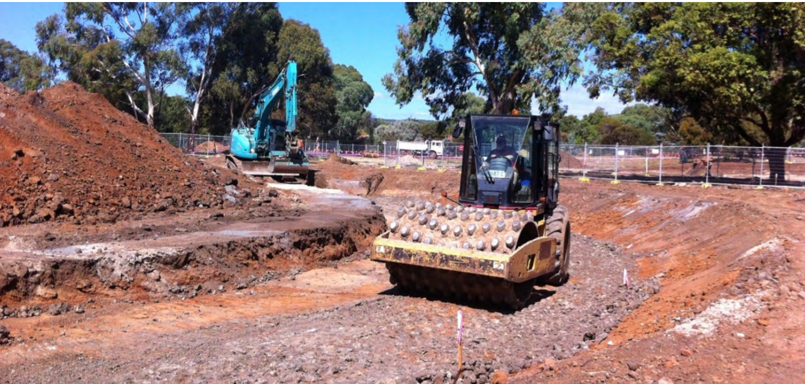
Figure 3.16 Installation of clay liner in a constructed wetland.
