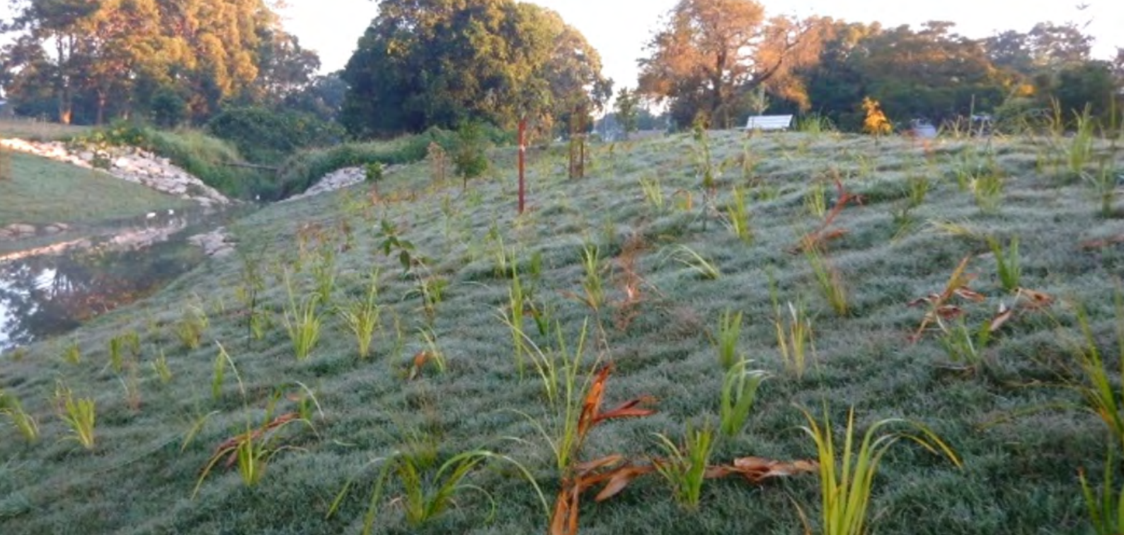
Figure 2.15 Turf in a bioretention system.
