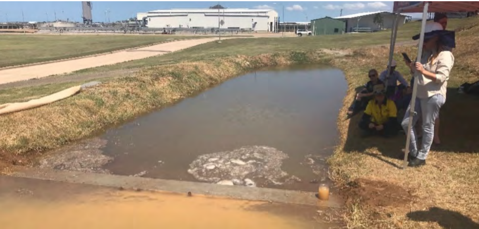
Figure 2.23 Use of a bioretention system as a HES basin during the building phase.
