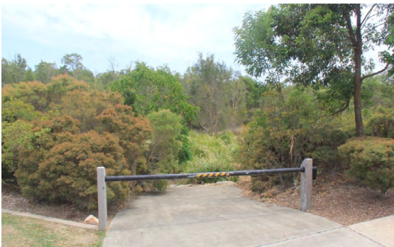
Figure 2.11 Maintenance access for a bioretention system.
