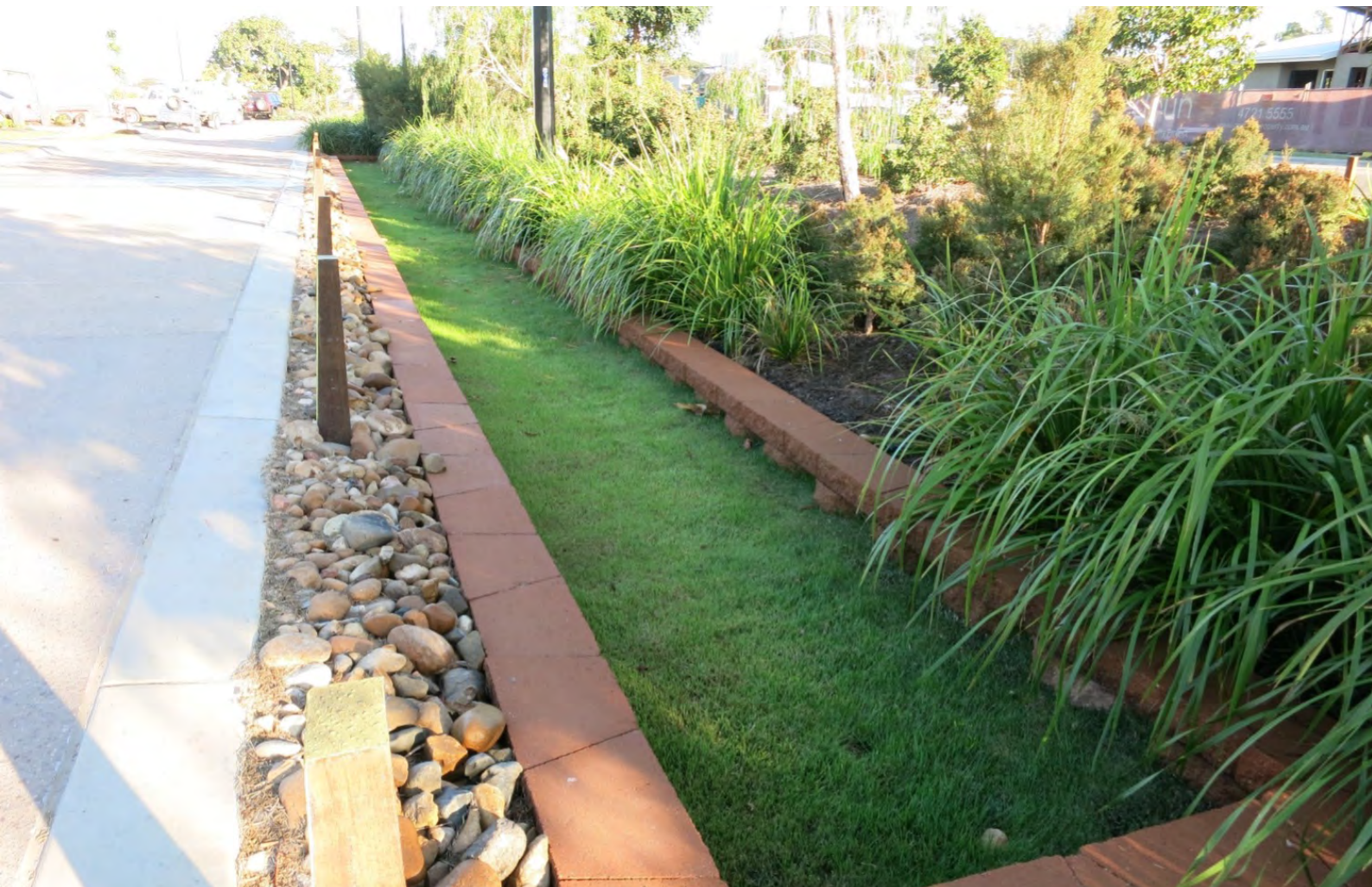
Figure 2.22 Temporary turf protecting a bioretention system.
