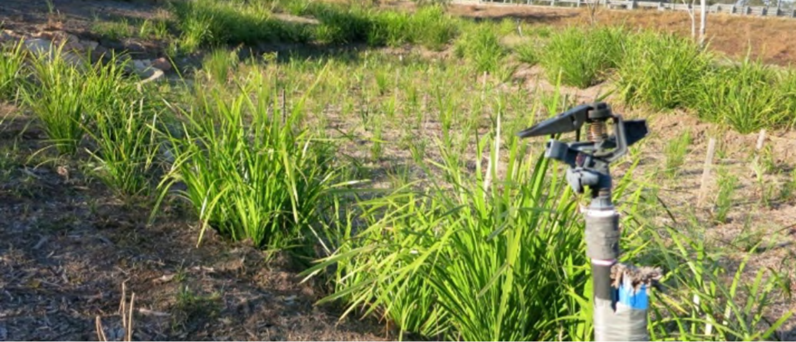
Figure 2.13 Temporary irrigation in a bioretention system.
