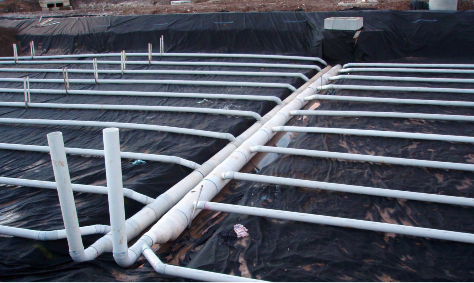
Figure 2.29 Under-drainage pipes in a bioretention system.
