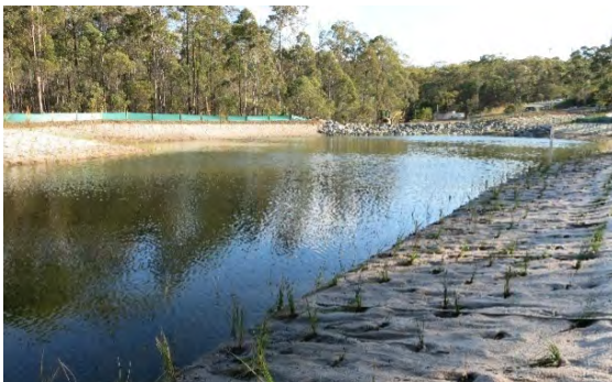
Figure 3.4 Erosion control matting in a constructed wetland.
