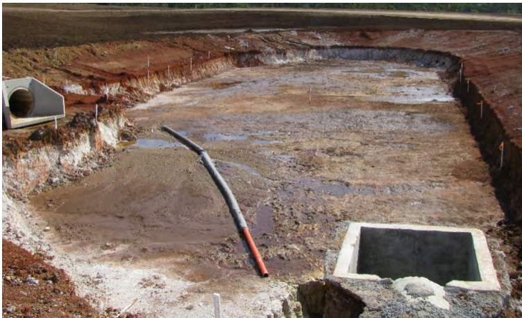
Figure 2.26 Bulking out a bioretention system.
