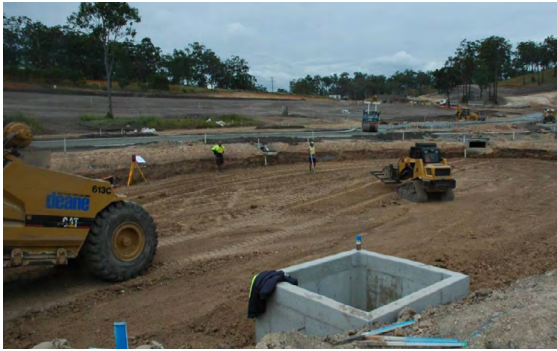
Figure 2.28 Trimming and profiling of a bioretention system.
