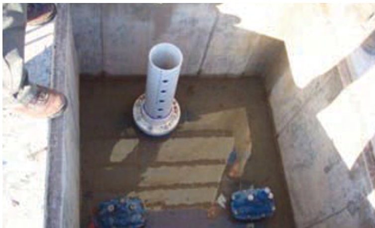
Figure 3.2 Outlet riser in a constructed wetland.
