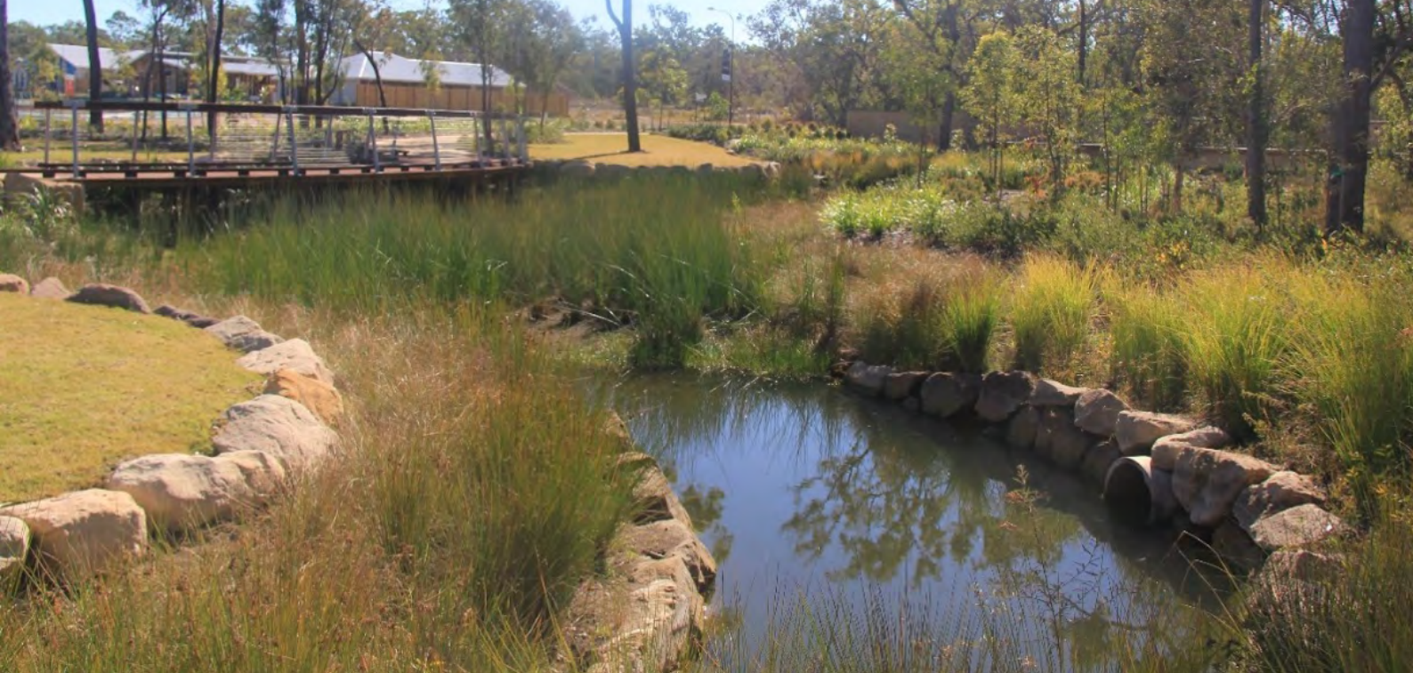
Figure 3.24 Established macrophyte zone of a constructed wetland.
