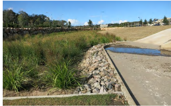
Figure 2.9 Rock apron downstream of a coarse sediment forebay.
