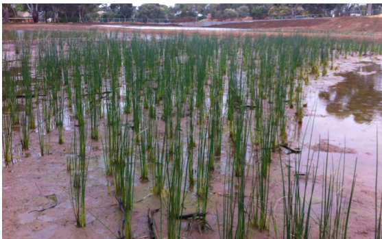
Figure 3.22 Plants installed in the mudflat environment of a constructed wetland.
