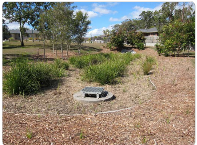
Figure 26: Immediately after rectification works
