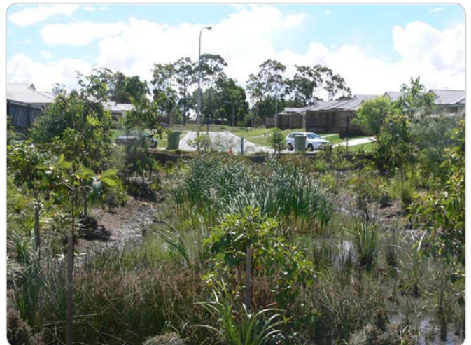
Figure 20: A System With Clogged Filter Media and Aquatic Weeds Requiring Rectification
