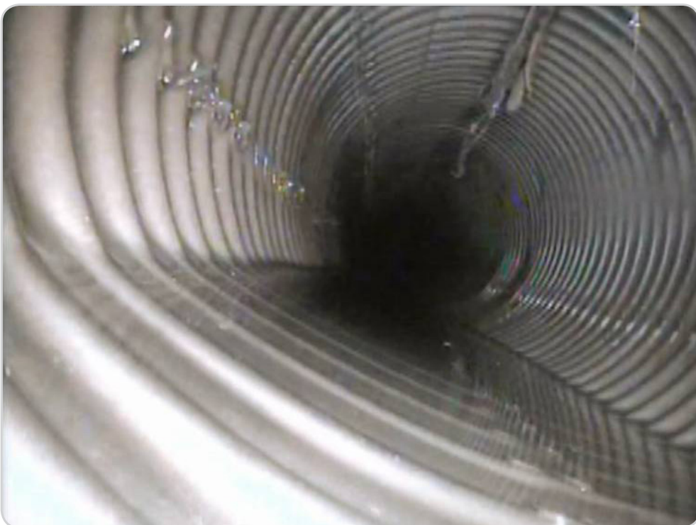
Figure 50: One of six underdrains showing only a few small roots in 2011
