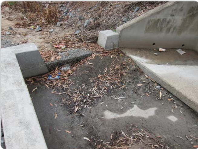
Figure 45: Coarse sediment from upstream building sites
