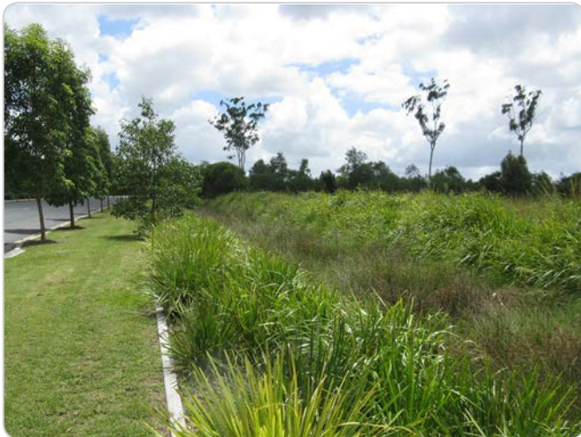
Figure 18: A System Ready for Maintenance
