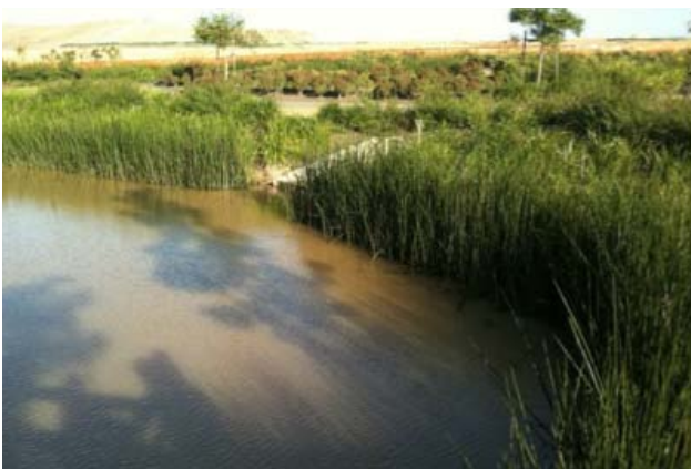
Figure 12 Example of properly functioning sediment basins
