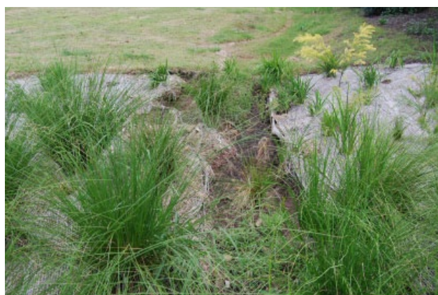
Figure 15 Erosion at the transition between wetland cells
