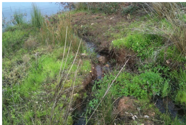
Figure 15 Erosion at the transition between wetland cells
