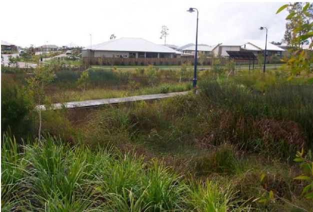
Figure 23: Constructed wetlands ready for final handover
