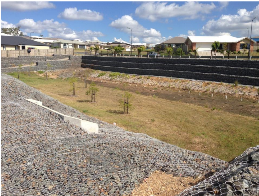
Figure 3. Examples of a stormwater treatment measure where function over-rides form
