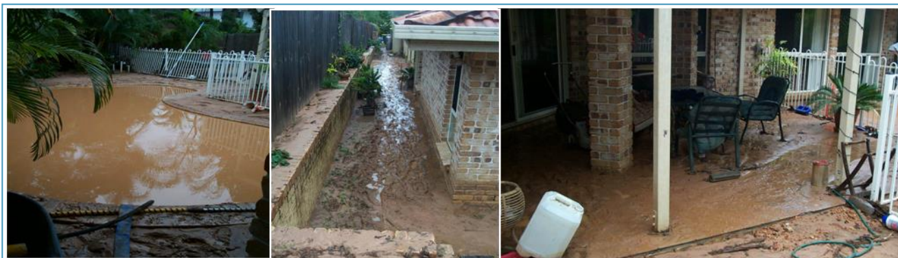
Figure 7 Impacts to neighbouring properties due to poor construction erosion and sediment control management
