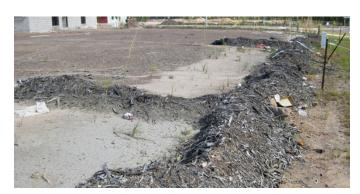
Mulch berm with upslope 'return' being used on small, flat house lots. (Source: Catchments and Creeks Pty Ltd)
