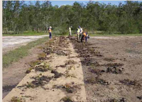
Installing the plugs. With geotextile on the left and without on the right.
