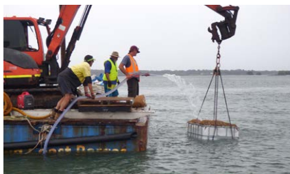
Deploying a shellfish reef array in the Pumicestone Passage.
