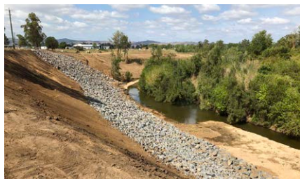
The finished rock wall revetment.
