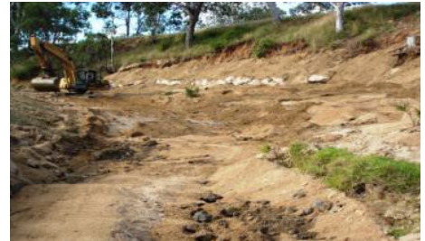
Stabilising the toe and retaining existing mature vegetation on the bank as well as regenerating vegetation in the early stages of establishment can form part of your plan.
