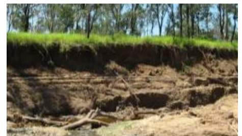
Bank scour occurs due to the action of flowing water removing soil from streambanks. Bare or poorly vegetated areas are especially prone.
