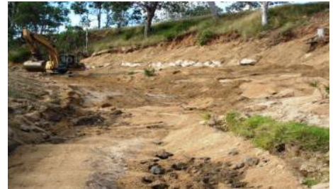
Stabilising the toe and retaining existing mature vegetation on the bank as well as regenerating vegetation in the early stages of establishment can form part of your plan.
