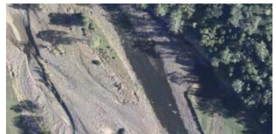
EAST HALDON: Scour has caused the stream to widen and the low flow channel to change course. Land used for grazing has been lost along with fences. Infrastructure on the floodplain has suffered impact.
