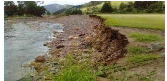
MT SYLVIA: Scouring has occurred here resulting in a very unstable steep bank, impacting on the productive potential of the farm.
