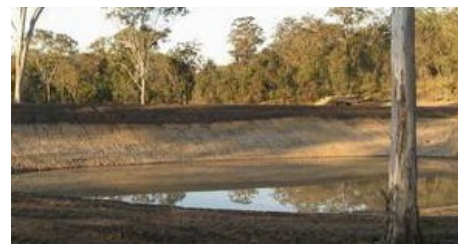
Drowning out a gully head by creating a dam can be a useful way to stabilise a gully.
