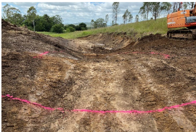
Figure 6. The gully sides were reprofiled to a 1:4 batter.
