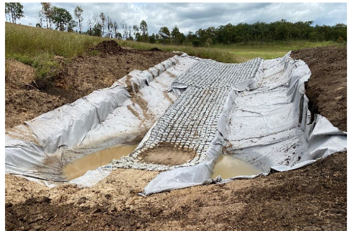
Figure 7. Geofabric overlaid across the entire chute and trenching and cement matting overlaid across the chute.
