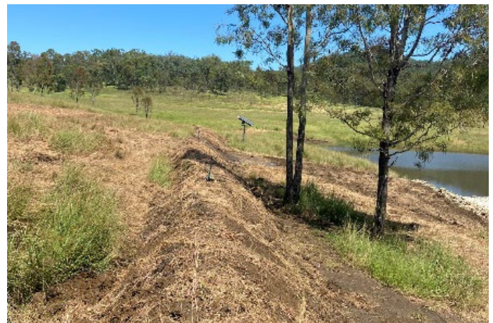
Figure 9. A contour bank was installed to divert runoff away from the restoration site.
