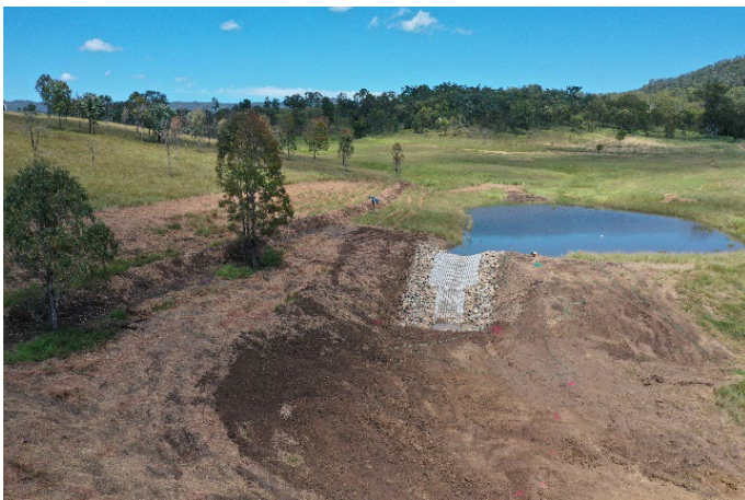
Figure 8. After construction the bare areas were seeded with a mix of productive perennial grasses and a cover crop.
