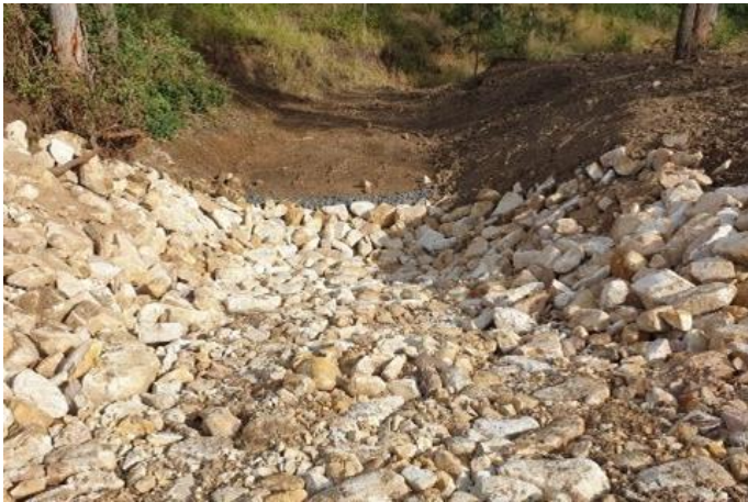
Figure 6. The rock chute after track rolling (looking downstream).
