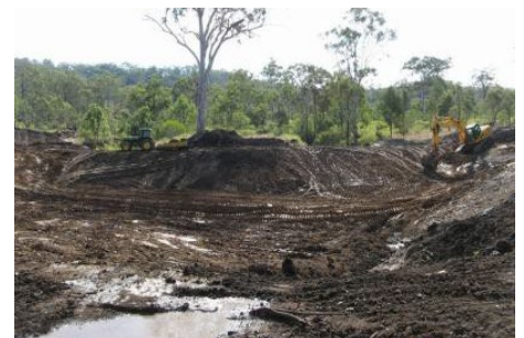
Constructing the control dam across the dual gully heads included compacting the soil to improve the structural integrity of the dam.
