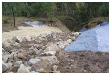
A rock chute was designed for the catchment size with an erosion control blanket built into the design.
