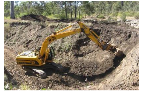
Battering the banks of the gully reduces mass failure and provides a platform for vegetation to establish to protect the soil.
