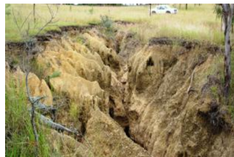
Disturbance to the soil surface and exposure of the subsoil to both rainfall and overland flow can lead to gully erosion.
