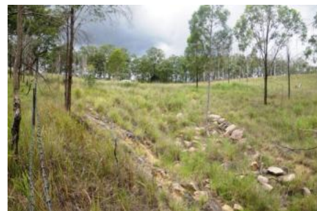
Topsoil spread over the rock chute aided the establishment of grasses that help hold the structure in place. It survived the 2011 and 2013 flood events.
