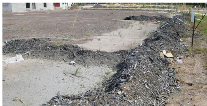
Mulch berm with upslope 'return' being used on small, flat house lots.
