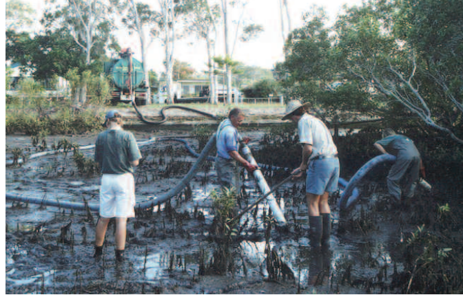
Removal of Lyngbya from mangroves using a vacuum pump.
