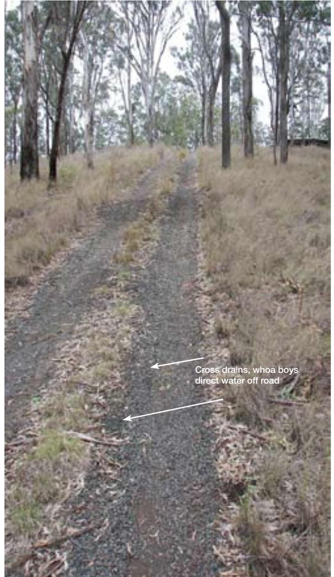
Basic erosion control – A steep track in the Helidon Hills area has been constructed on a ridge line with cross drains (whoa boys) to take water off the road to reduce erosion.
