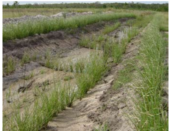
Vetiver hedges planted across the drain and along its banks have slowed the movement of water and trapped sediment on the drain floor (above).
