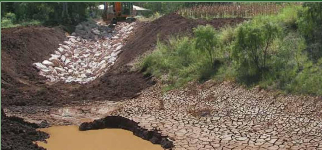
**SEOC Sediment Pond and Gully Erosion Repair** Heavy rainfall can cause an immense volume of water to flow through gullies and as overland flow in the Lockyer Valley. Siltation ponds prevent further sediment from entering the main channel. This sediment pond is being repaired so it may cope with future storms.
