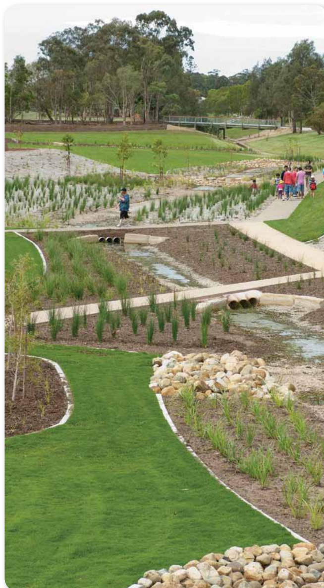
Fitzgibbon Chase - Water Sensitive Urban Design Project and winner of the 'BP-Water Sensitive Urban Design Award' at the 2012 Healthy Waterways Awards.
